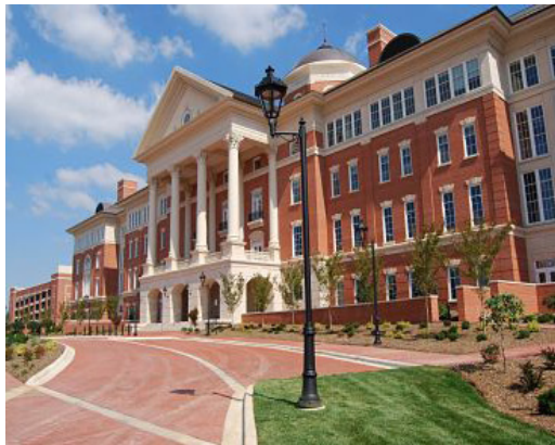
DAVID H. MURDOCK CORE LABORATORY BUILDING
